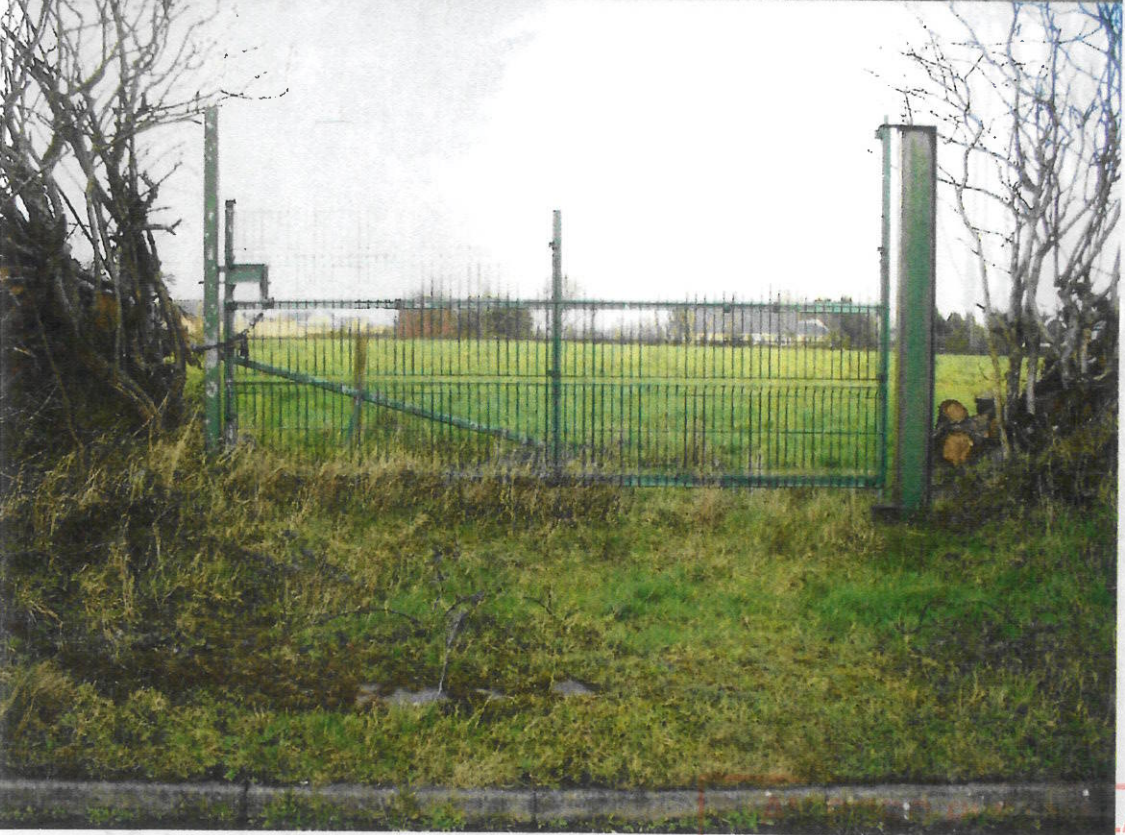
Gate A. Height of top of gate over ground level = 1.7m. Height of gate posts = 2.25m
